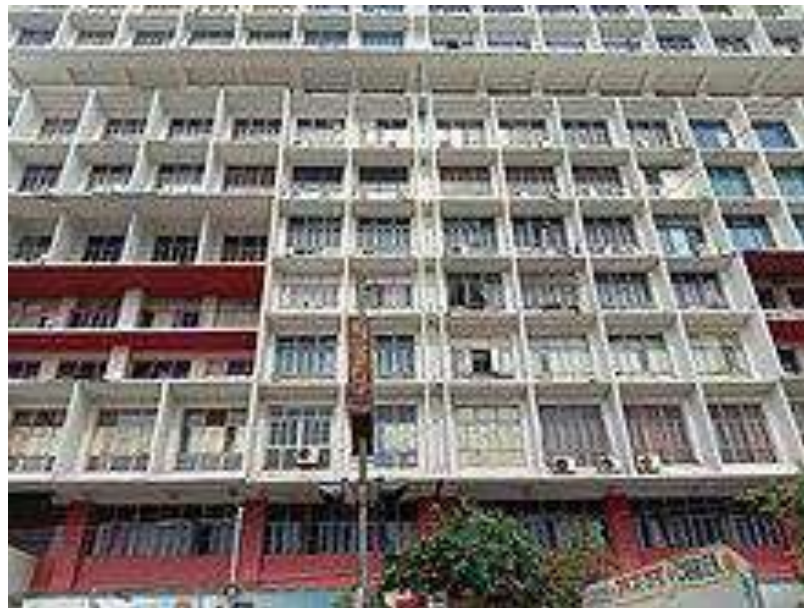
Yogayog Bhawan (head office of the West Bengal wing of India Post), at Chittaranjan Avenue, Bowbazar, Kolkata.
